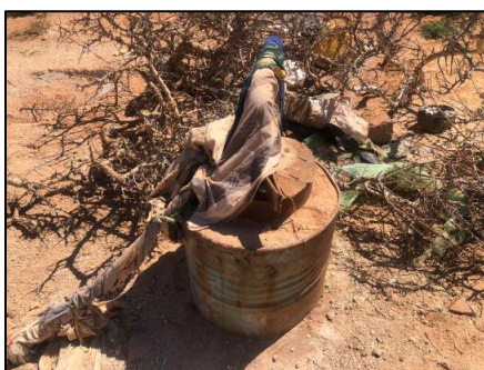
Broken borehole in Guumeys, Sool (Photo: SRCS)
