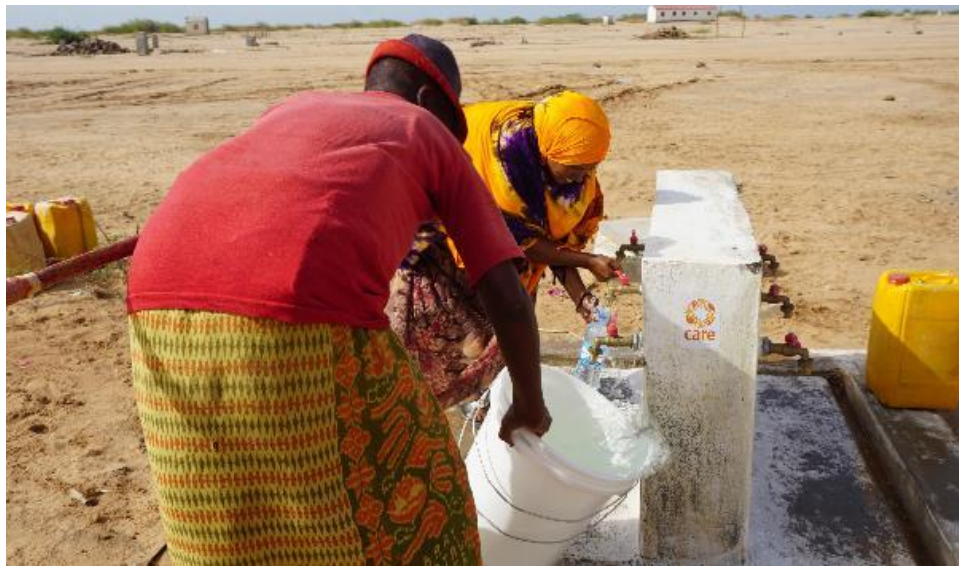
Figure 4.4.1.1: School and water supply facilities damaged in Ceelsheikh
